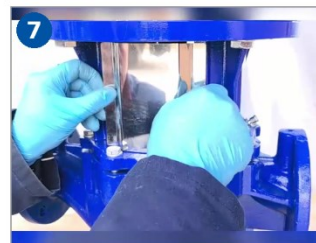
Refit the coupling-guard plates
